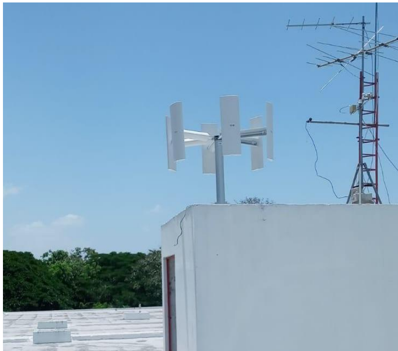
Fig 9 – Installation of Wind Turbine
