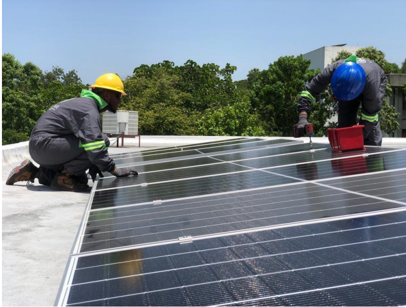
Fig 8 – Installation of the 3KW PV System
