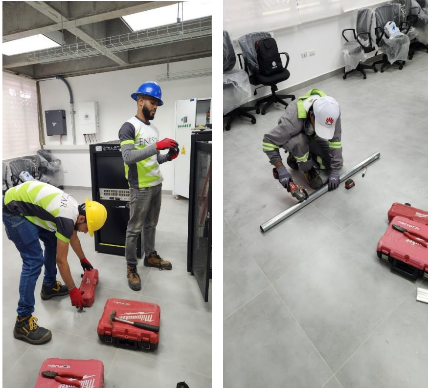
Fig 13 – Technicians installing the remaining electrical wiring and conduits
